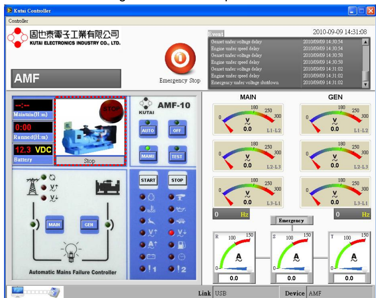
Figure 5-3 State of generator
